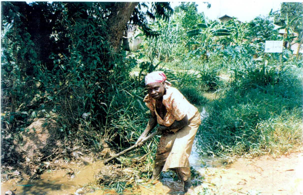
BDEA member clearing a drainage
